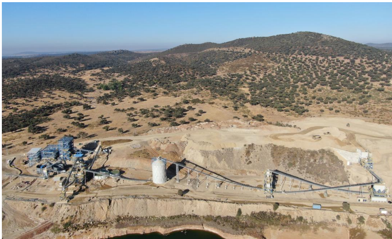
Figure 2. La Parrilla construction nears completion
